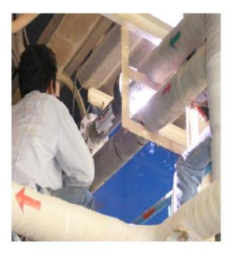
The MagCat was installed after the pump and was treating pipework 1/2 km in length.
