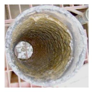
The thickness of scale inside the pipe was an average of 10mm decreasing the flow. The scale had also increased the weight of the pipe and, with much of it being installed on the ceiling, there were concerns that it could become unstable with the potential danger of it collapsing.
