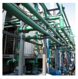
**B-2** Water pump 22 Kw , 30 HP , pipe diameter is 4 inches. The water flow rate is 45 M3 / Hr. or Flow velocity is 1.54 m/ sec.
