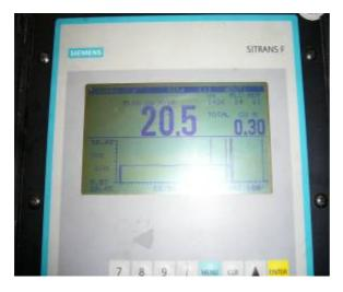
A-5 Flow rate of cool water was 20.5 M3 / Hr and / or A-6 Flow rate of hot water outlet couldn't detection
