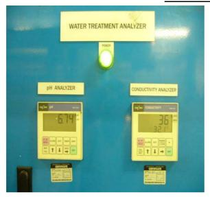
C-1 Cool water analysis at Area-2pH = 6.74 , Temperature = 32.1oCConductivity = 36.1 µscm
