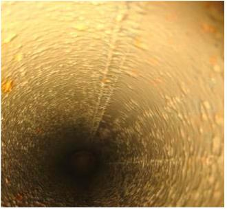
Picture of scale inside pipe after installed CAT -100
