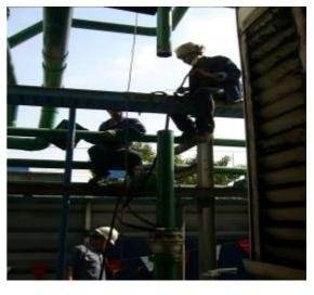
B-4 The pipe was cut above the pump 2.00 meters
