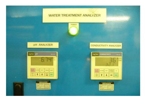
Further to an above data of analyzer, cool water have been proofing a good qualities however there are having a deposit scaling inside pipe and heat exchanger. The mechanism of these factors are
