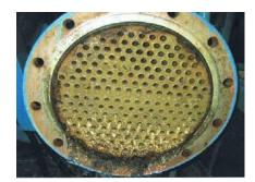
Compressor after cooler with scale
