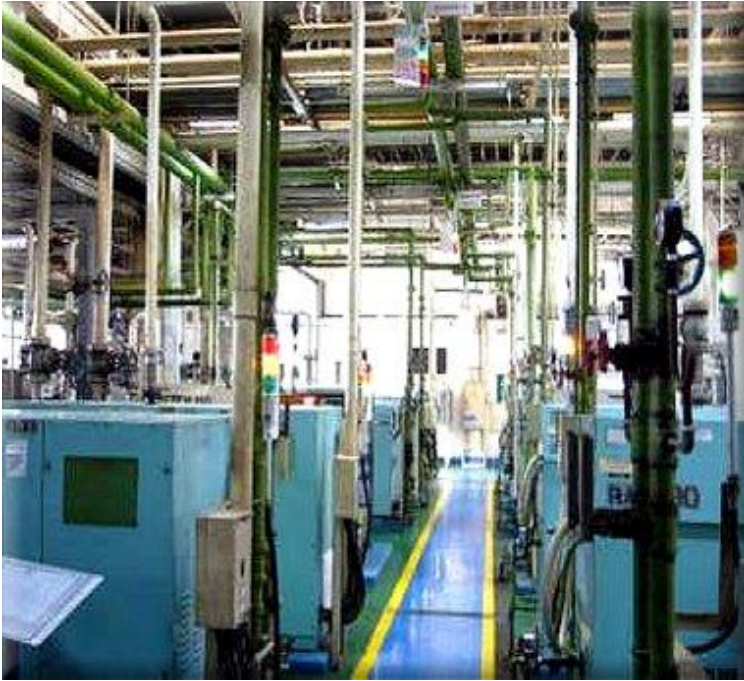
Compressors & Air Dryers at Thai Honda
