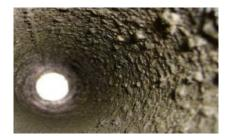
Feed Line to compressors with scale deposition
